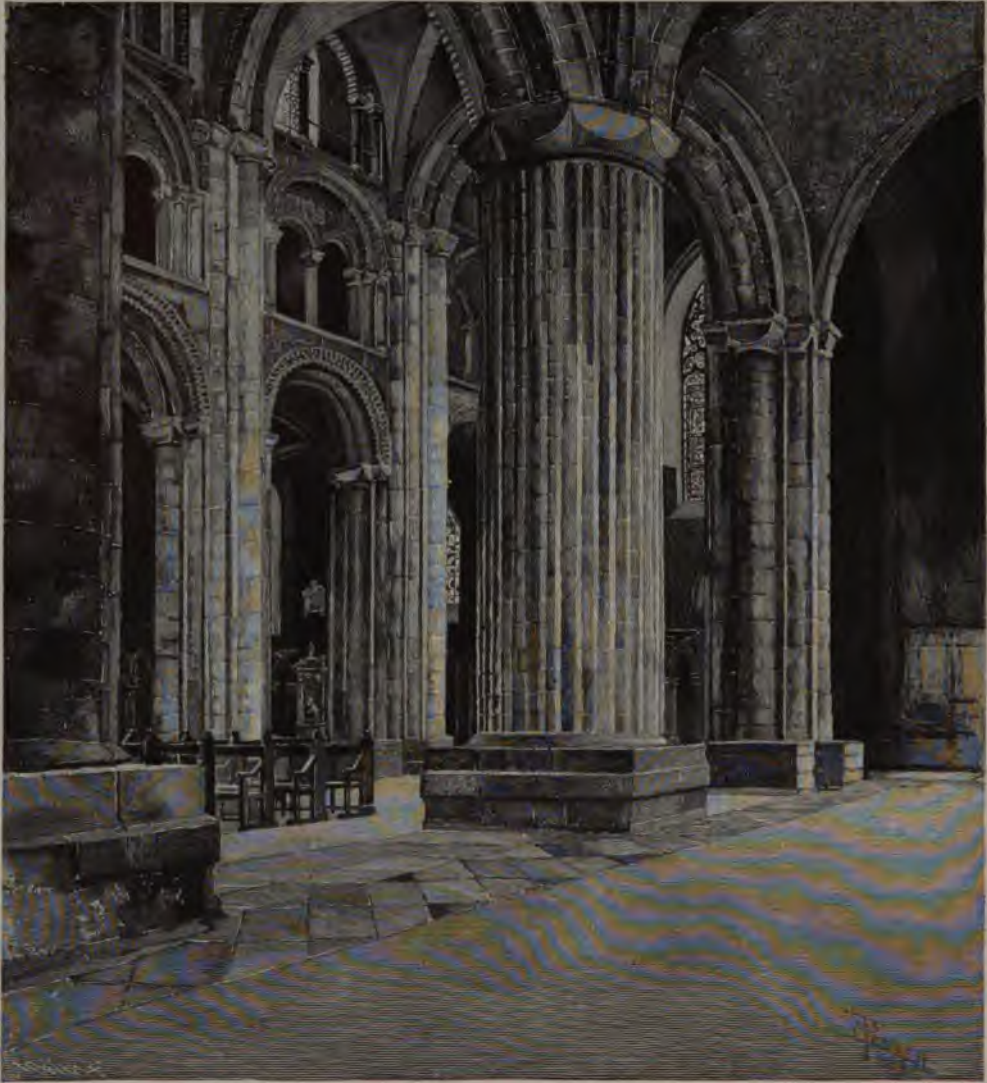
THE WEST END OF THE NAVE, FROM THE NORTH DOOR.
